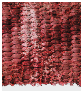
Heavy soiling / mold
