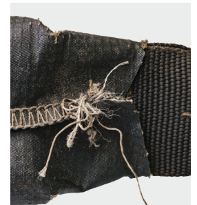
Ripped / missing stitching
