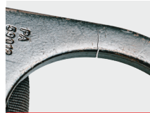
Cracks in D-ring or fasteners
