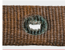
Grommets not secure (wiggling) or missing
