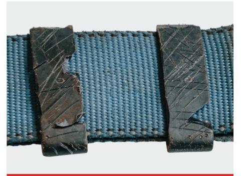
Loose / damaged mountings
