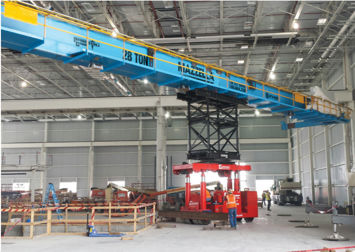
Heavy, long span double girder crane installation using a “tri-lifter”.
