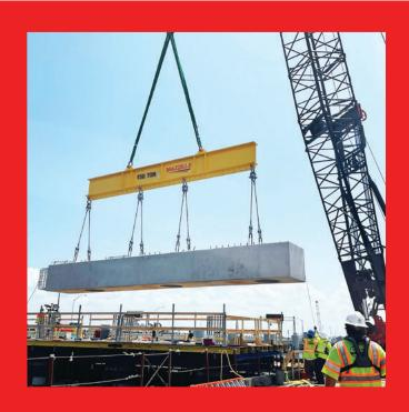
Mazzella is a leader in the design and development of custom engineered below-the-hook lifting devices and lifting attachments for use with all types of cranes.
